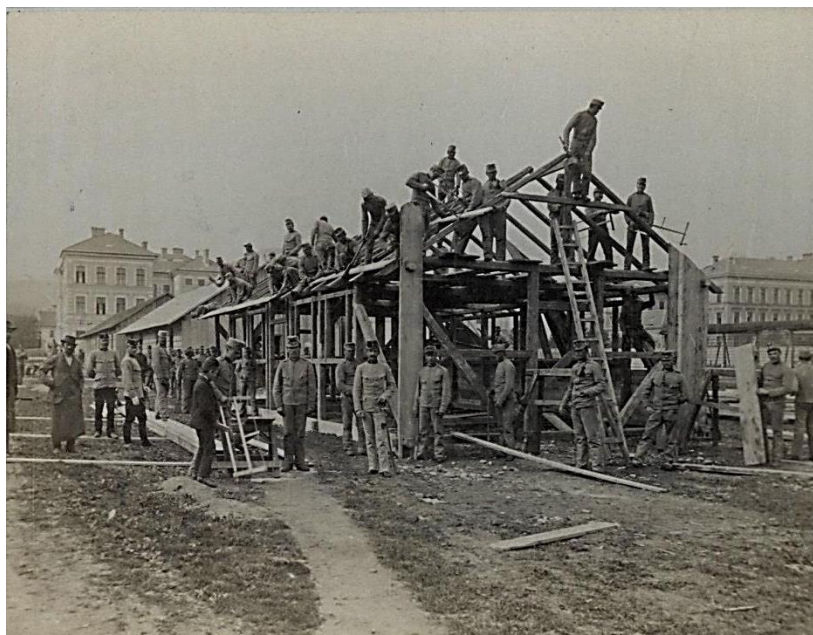
Soldiers building barracks. Photo by W. Helfer
