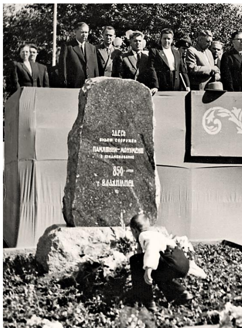
Laying the foundation stone of the monument in Svoboda square Source: Naslediye Vladimirskoy oblasti [Vladimir Oblast Heritage], https://vk.com/wall-213594879_298
