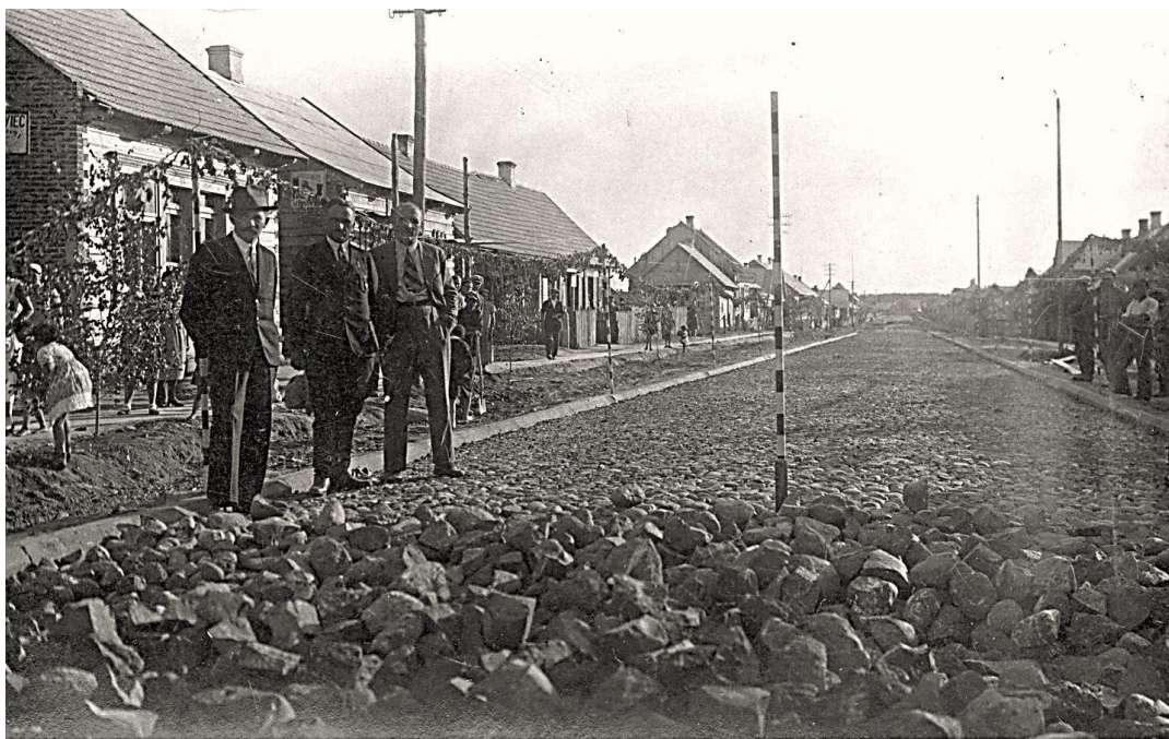
Construction of a street in the city of Ivatshevichi, Polesie Voivodeship
