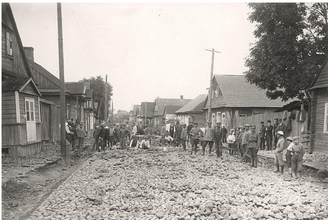
Paving Jozef Pilsudsky Street in Novogrudok
