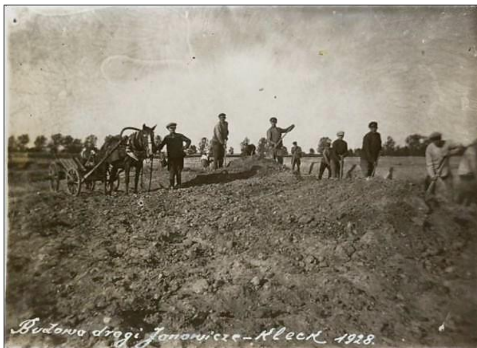
Construction of the Klets–Yanovichi road, Nesvizh powiat of Novogrudok Voivodeship, 1928
