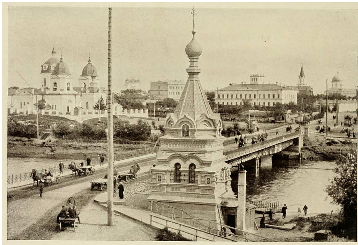
Omsk in 1914. View of the Iron Bridge
